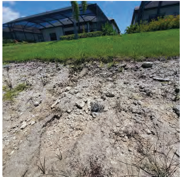
Photo #68 Minor erosion near the bottom of the lake slope
