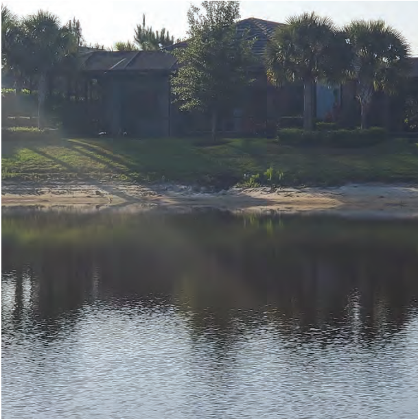
Photo #30 Minor erosion near the bottom of the lake slope
