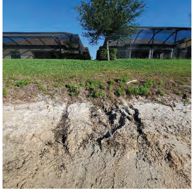
Photo #35 Minor erosion near the bottom of the lake slope
