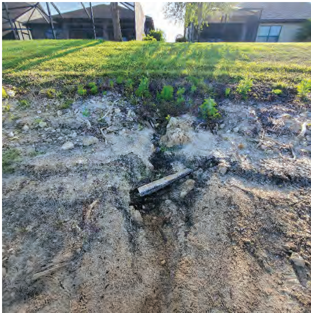
Photo #34 Minor erosion near the bottom of the lake slope
