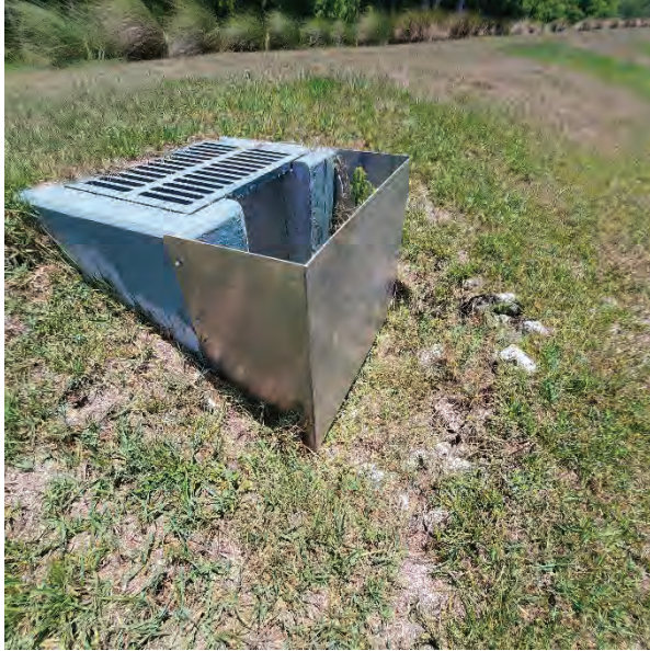
Photo #65 Control Structure in Lake 1-5
