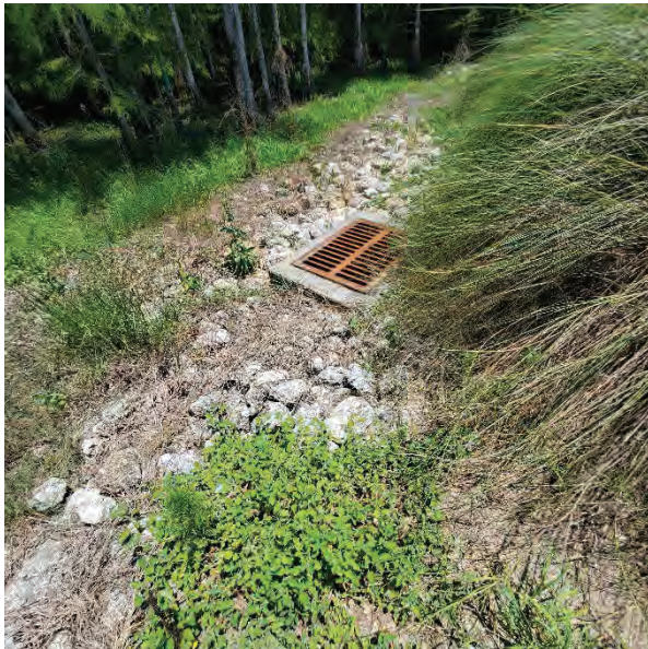
Photo #66 Control Structure in Lake 1-5
