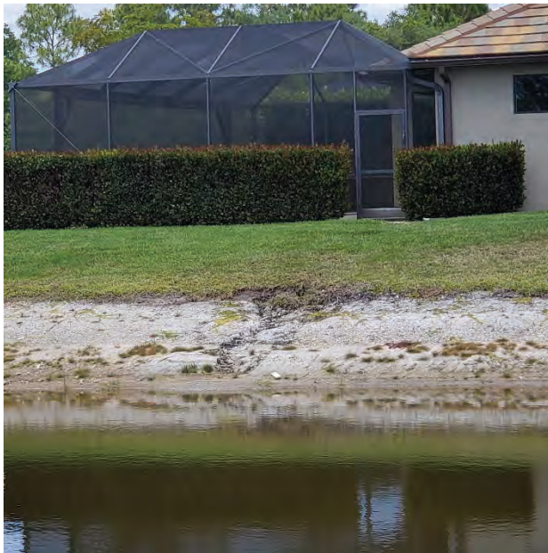
Photo #22 Minor erosion near the bottom of the lake slope
