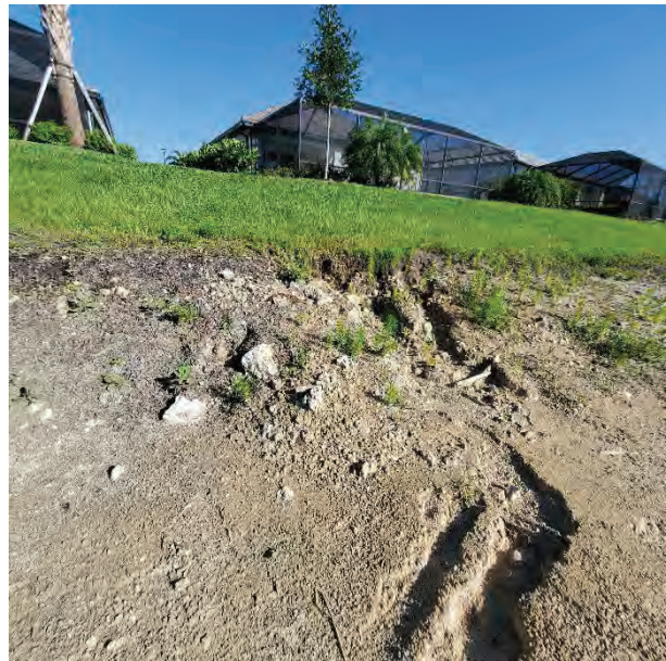
Photo #36 Minor erosion near the bottom of the lake slope
