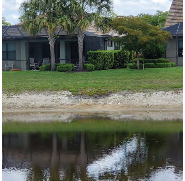
Photo #23 Minor erosion near the bottom of the lake slope
