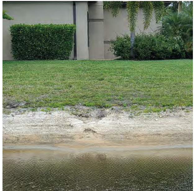
Photo #24 Minor erosion near the bottom of the lake slope
