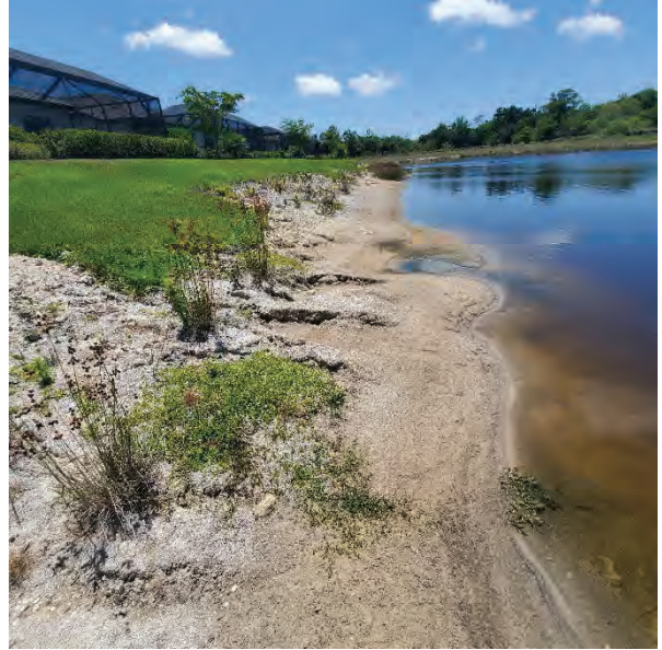
Photo #67 Minor erosion near the bottom of the lake slope
