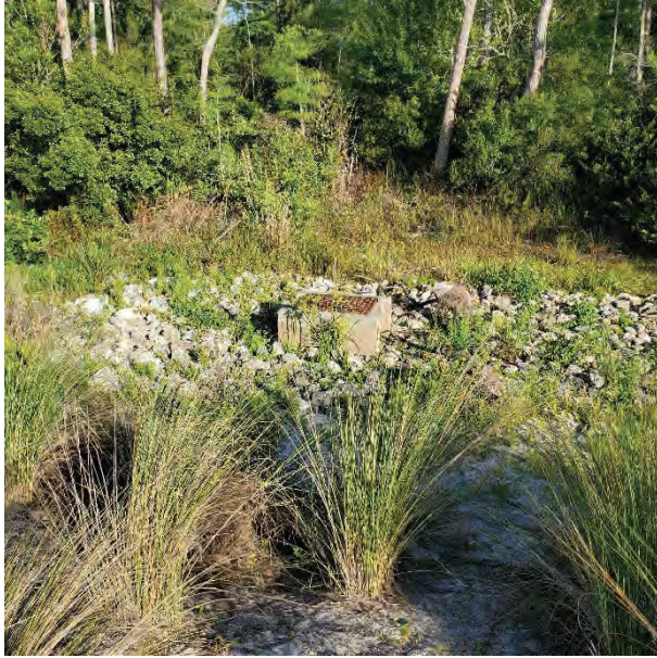
Photo #33 Control Structure in Lake 11-6
