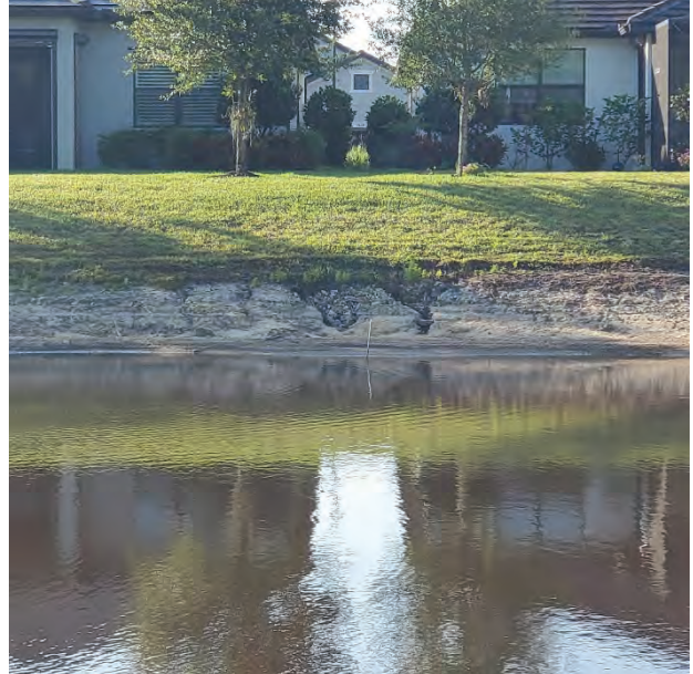
Photo #31 Minor erosion near the bottom of the lake slope
