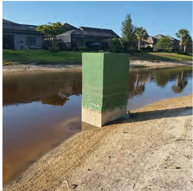
Photo #32 Control Structure in Lake 11-6
